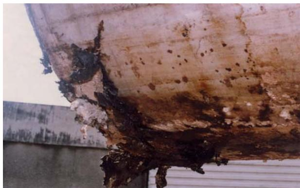
Fig. 4 Pitting Corrosion of the Decay Tank Bottom
